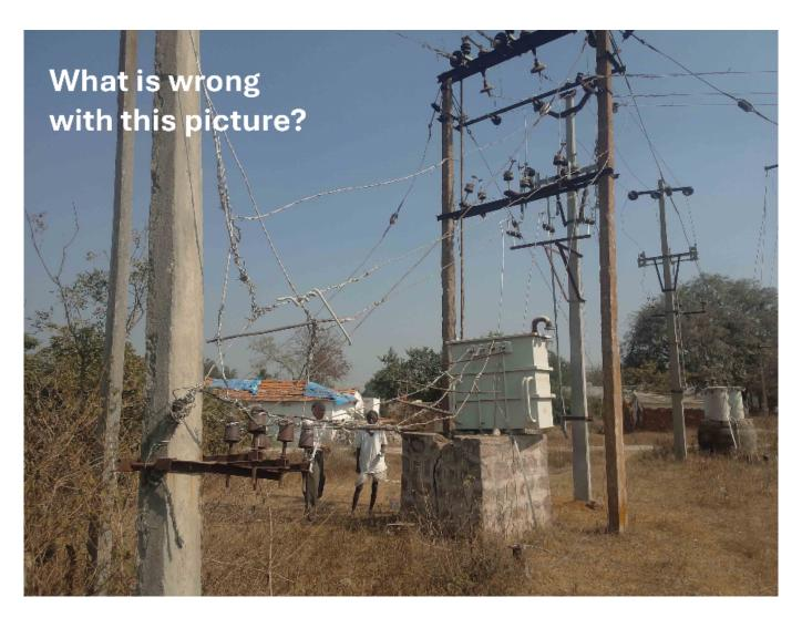
Example of poor quality, failing equipment and the danger it represents (Photo credit: C. Satish)
